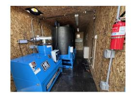
systems installed within Hydrosite are individually ETL certified to UL1776, UL979, CE and CSA safety standards. Hydrosite containerized equipment room, as an entire system, is also ETL certified to UL1776, UL979, CSA and CE.
